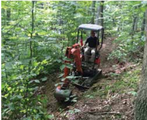
NPS staff, trail crews, and contractors use specialized mountain bike trail equipment to build a smooth, sustainable trail.
